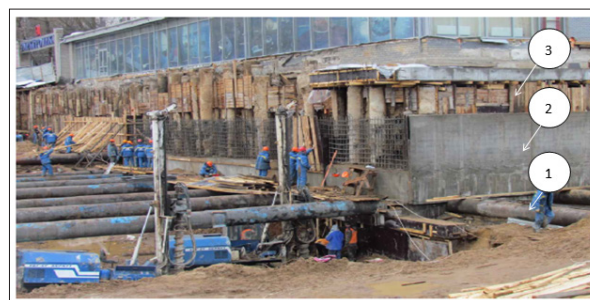
Figure 1: Geotechnical works at node "1" to strengthen the deformed existing retaining wall of the construction pit enclosure: 1-steel pipes with a diameter of 1000.0 mm as bunkers; 2-monolithic reinforced concrete buttresses; 3-construction pit enclosure (bored injection piles, filler made of 50.0 mm thick boards).
