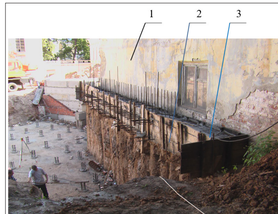
Figure 3: Retaining wall made of two rows of bored piles ERT (RIT, FORST, ERST) as a pit enclosure in Nizhny Novgorod: 1 - reinforced object; 2 - pit enclosure made of two rows of bored piles ER T (RIT, FORST, ERST); 3 - monolithic reinforced concrete strapping belt
